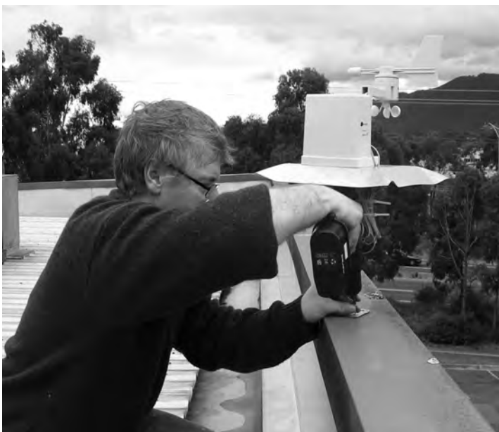
Figure 13-2. Weather station sensors and transmitter being installed
